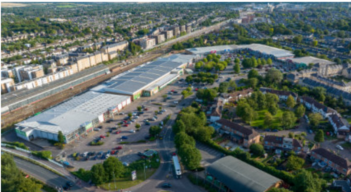
North aerial view towards Beehive Centre
